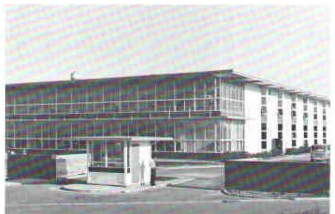
Yokogawa-Hewlett-Packard plant, making extensive use of glass walls, is light and airy inside. Building is located 30 miles from Tokyo.
