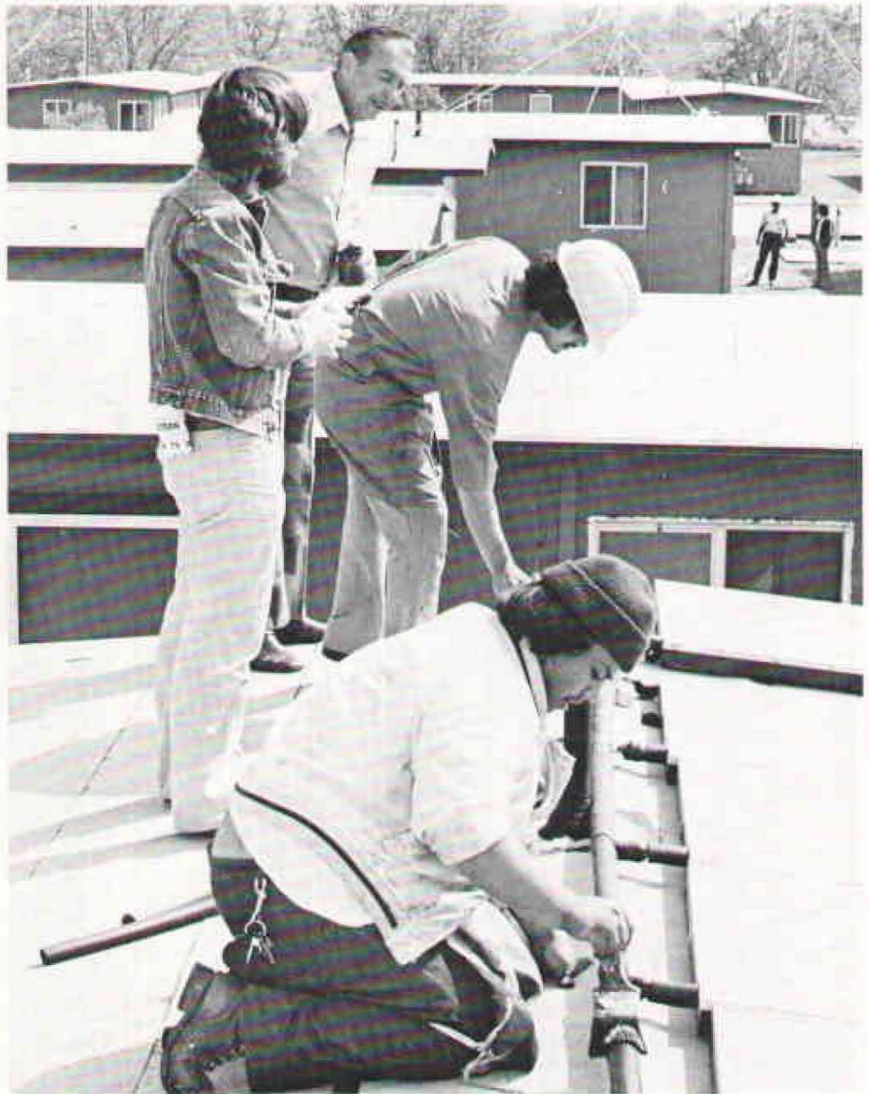
Mac McFee (top center) coaches solar heating class.
