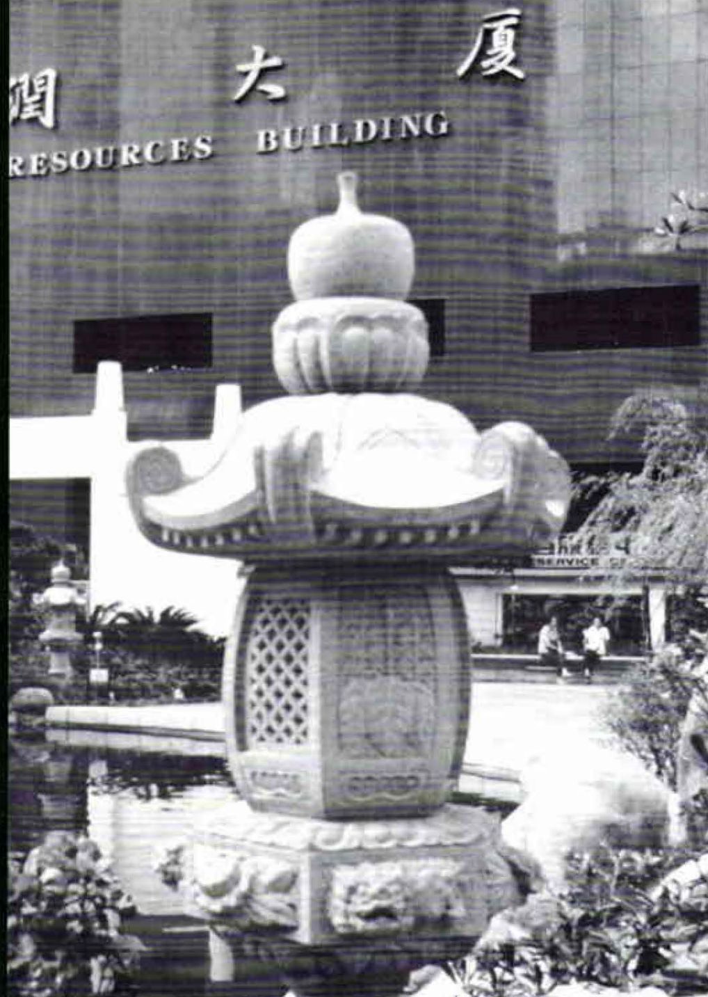
Building in Hong Kong. Both HP Hong Kong and HP Asia are feeling the brain drain.
