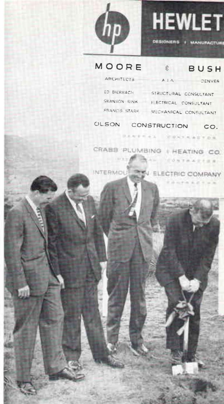
Bill Hewlett did the ground-breaking honors as construction of HP's new Colorado Springs plant officially got under way August 12. Kibitzers include (left to right) Curt Van Rensselaer, general manager of the Oscilloscope Division, Harry Hoth, mayor of Colorado Springs, and Dave Packard.
