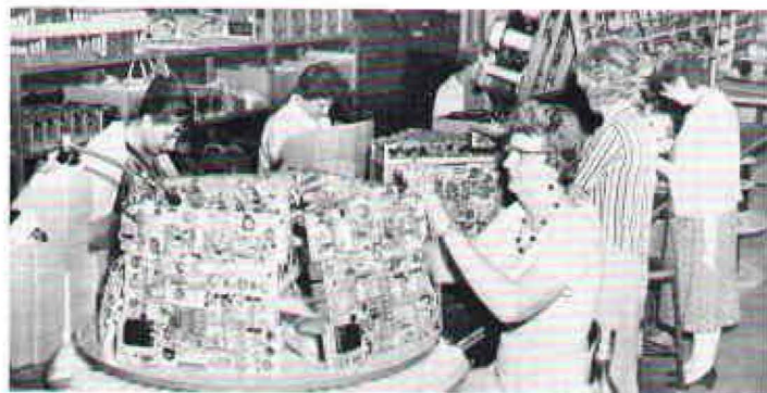
ABOVE: Modern production lines utilize "lazy Susans." Women here are assembling FM stereo modulators. BELOW: George Sanford demonstrates application of a BRC FM-AM signal generator with a Dymec servo programmer. System reduces tedious calibration to a push-button operation.
