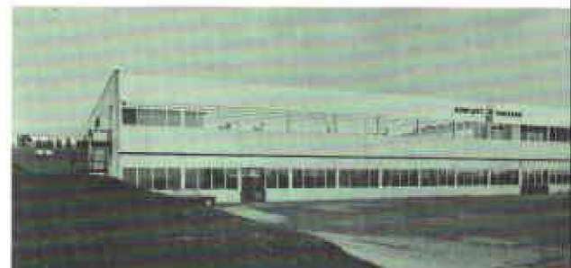
New building at Boeblingen brings total plant area to 80,700 square feet.
