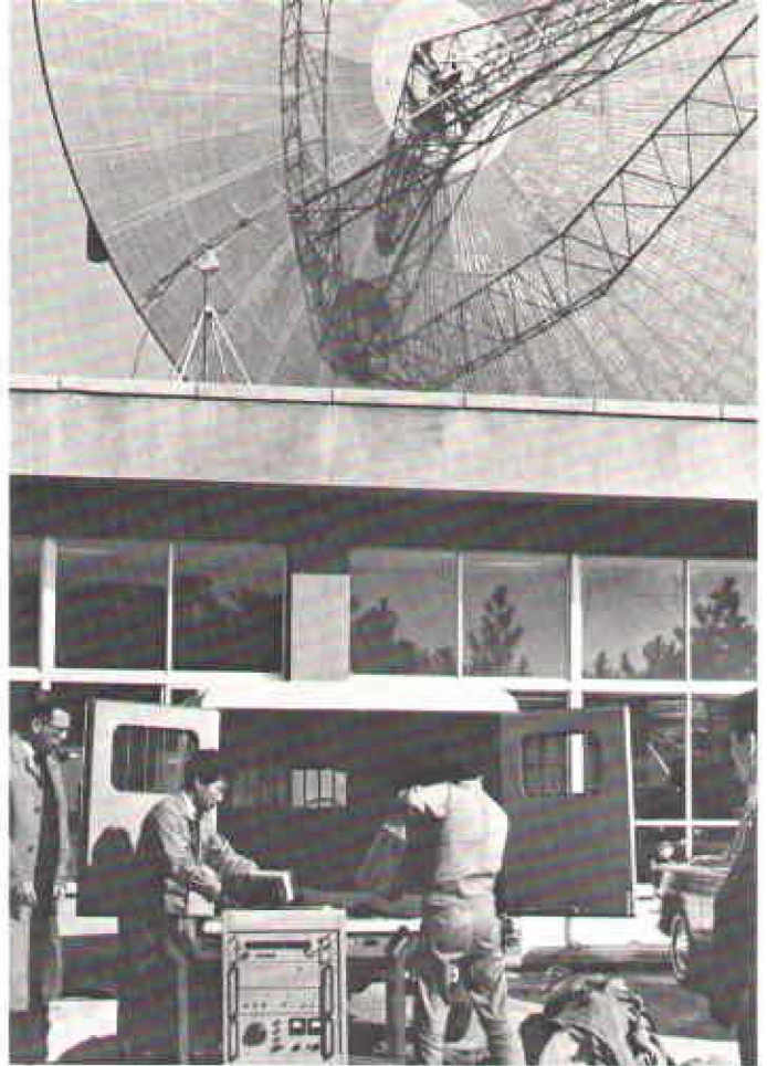
The flying clocks, with their HP cesium beam standard "atomic hearts," are unloaded at Koshima, Japan, preliminary to U.S. Navy project of synchronizing U.S. time with that of Japan.
