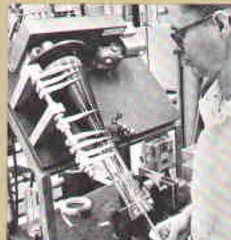
A cathode ray tube turns slowly on special equipment as Lee McLaren applies a conductive coating to the inside of the tube.
