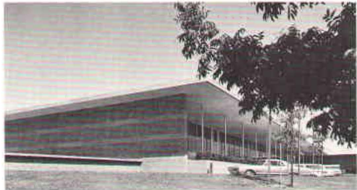
PALO ALTO — Completed in June, this new 30,000-square-foot addition to the headquarters complex in Stanford Industrial Park provides substantially more space for HP Laboratories, the corporate research and development group. Known as Building 1A, it is occupied by a staff of 200.
