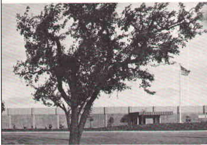
MOUNTAIN VIEW, CALIFORNIA — Delcon Division and Customer Service Center employees occupied their new 65,000-square-foot plant (at left) during fiscal 1967. The exterior features sandblasted panels of concrete with exposed creek pebbles. Twin building on the right was occupied by the Mountain View Division during fiscal 1966.
