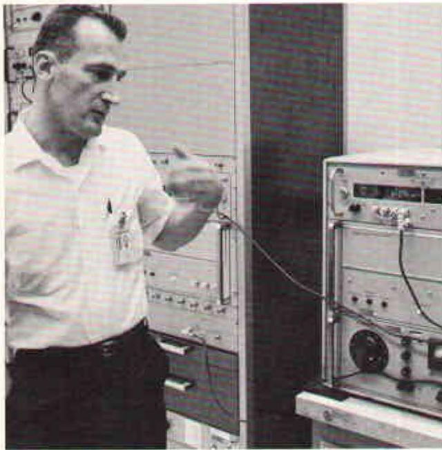
Fuzie, head of JPL standards/calibration lab at Goldstone, discusses role of HP atomic clock in synchronizing timing throughout Apollo network. All worldwide facilities must sync within very few milliseconds.
