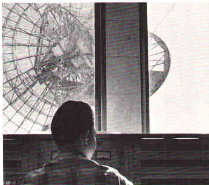
Operations room of Apollo-Goldstone tracking station was in direct contact with Apollo 8 during the most critical phases of the journey via the 85-foot antenna above. The station, a key site in NASA's worldwide network of Apollo facilities, houses approximately 160 six-foot racks of electronic gear.
