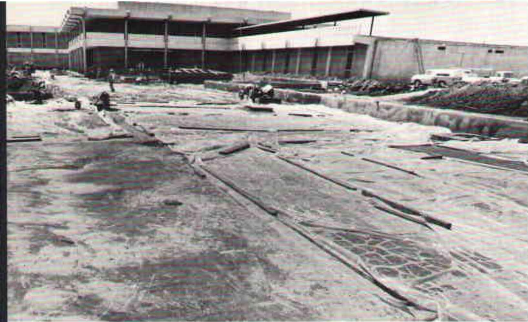
Photographed in early June, first phase of new Santa Clara Division plant still had several months to go in construction although portions were occupied and in operation by large contingent of people from former F&T. Foreground will become a large reflecting pool providing a secondary water supply for fire protection as well as an attractive setting. Eventually the roof will become a recreational patio. Exterior walls feature precast concrete panels faced with brown-hued crushed rock.
