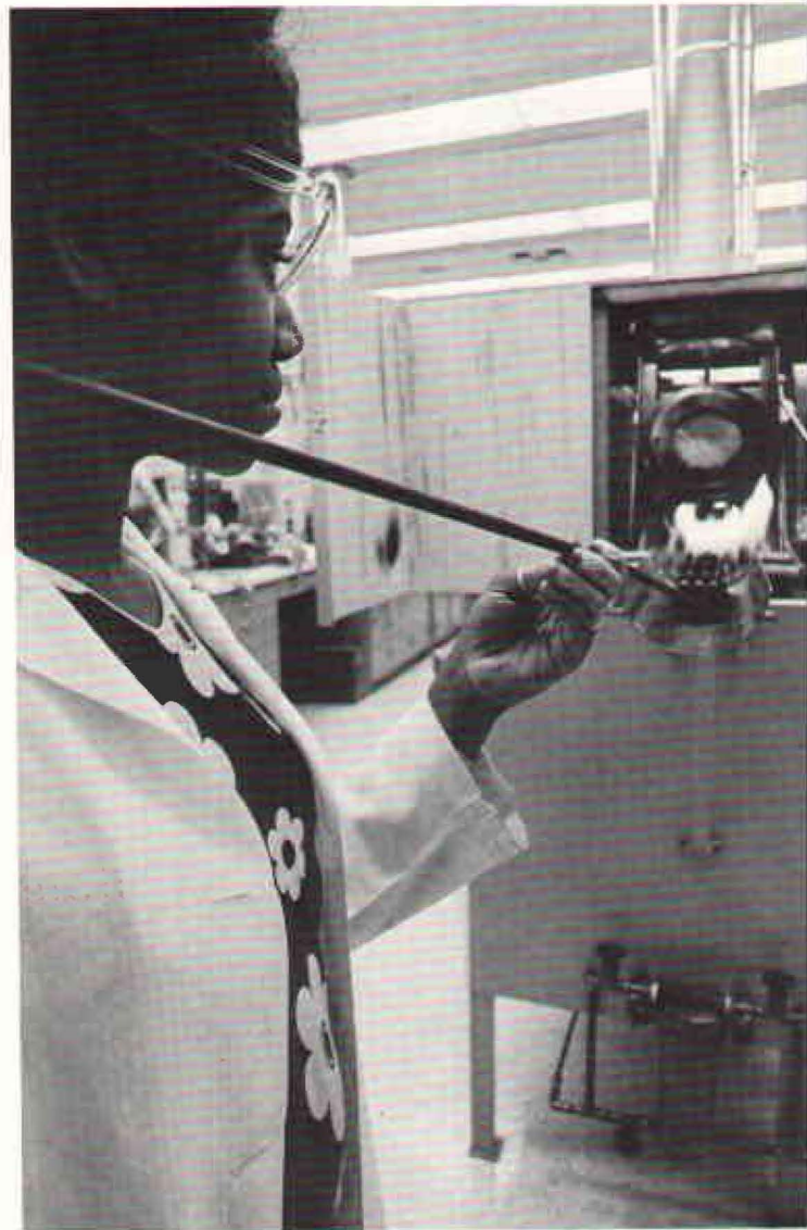
Object of glass-to-metal bonding process is to create hermetic sealing that will contribute to the very long life expectancy of HP microcircuits. Here Paula Clarin loads a completed 'boat' of amplifier frames into furnace for sealing. Later each package frame will be combined with other package elements plus a microcircuit to form the completed component.
