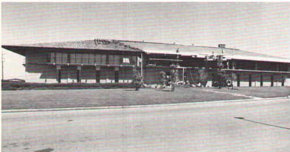
Until a few months ago this International Operations headquarters in Stanford Industrial Park represented the first half of a total building design. It was purchased that way in November, 1967 from a publishing company. Now the design is being carried out to its full size of some 25,000 square feet, to provide much needed space for International's global growth.
