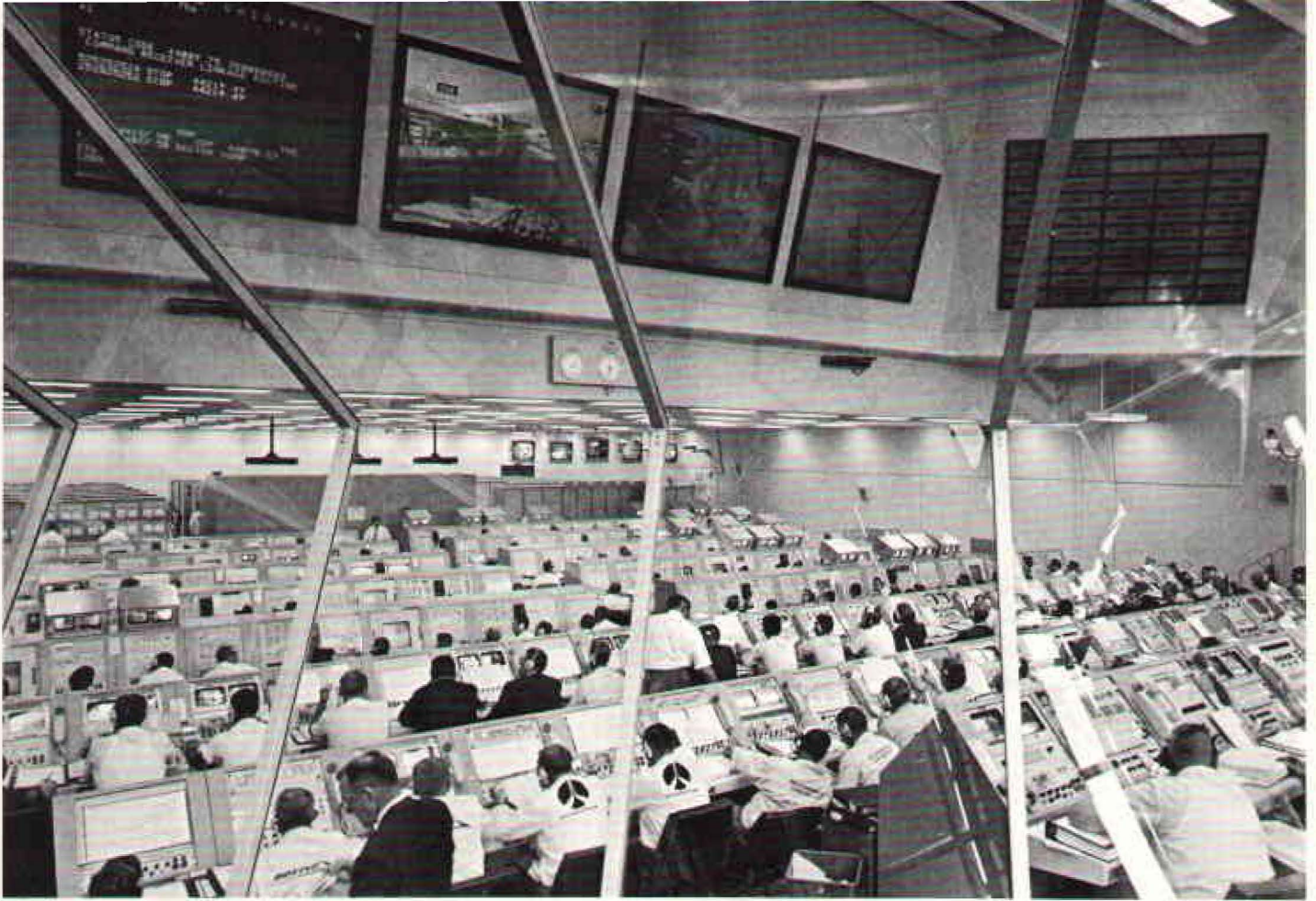
Launch Control Center at Cape Kennedy, shown here, and Mission Control Center at Houston both were equipped with a wide range of HP gear for communications systems and calibration facilities. The New Jersey Division, for example, provided precision picture monitors, power supplies, FM-AM telemetering signal generators and RF vector impedance meters.
